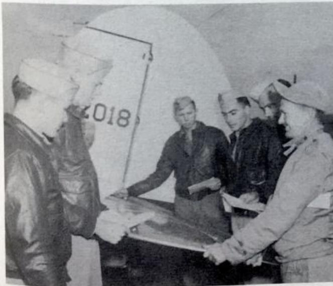
In combat a pilot is often his own mechanic and crew. He must be able to make quick repairs with the material at hand. Here the grinning sergeant shows how to patch a punctured stabilizer.
