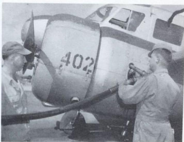
On the flight line an A.T. 17 is carefully serviced before flight. Planes take off with full tanks on all hops, require unceasingly vigilant care.
